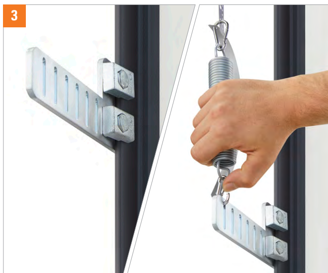
3 At the shaft pit: Fit the rail mounting. Hook the tension spring and securing band into the snap hook and connect to the rail mounting (same slot as in shaft head). Cut coded band to length and use the snap hook to connect it to the tension spring and securing band.
