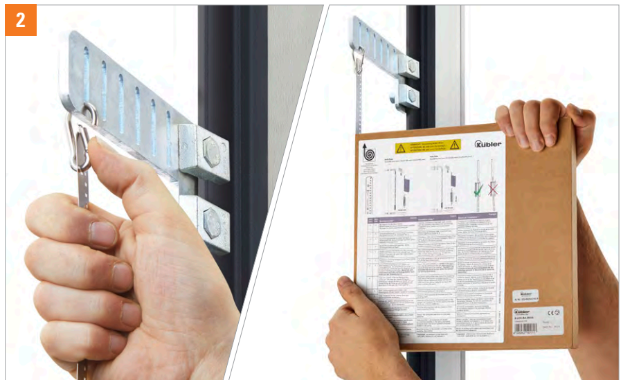
2 Use the snap hook to hang the coded band into the slot of the rail mounting. Be careful with the lateral alignment of the holes in the coded band. Follow the illustration on the name plate of the sensor. Follow the installation instructions on the coded band packaging (in 6 languages). The coded band unrolls from its cardboard packaging during downward travel.
